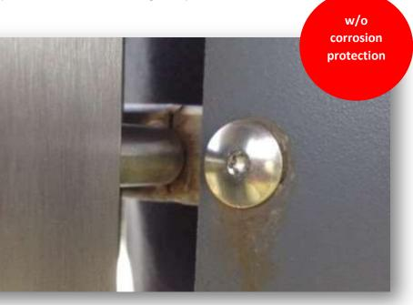
Similar damage patterns in coastal areas are also found in the area of aluminium rivets for fastening façade panels to aluminium substructures (white rust). The illustration shows the fastening of HPL façade panels with stainless steel rivets on a stainless steel sub-construction.
