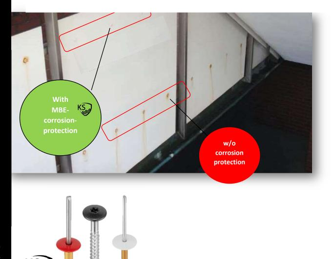
MBE offers specially protected fastening elements for affected regions (from coastline up to 50 km). Order fasteners for certain areas with MBE-Corrosion-Protection.
