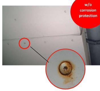
Since it has long been known that stainless steel is not (always) corrosion-free, for some time now people have been talking about corrosion-resistant stainless steels and fasteners in many areas. Stainless steel fasteners affected by brown staining are usually not completely destroyed, but a permanent surface damage may remain.
